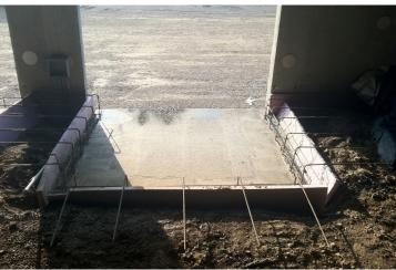
Concrete pads are poured. The pads must be sufficiently thick and strong enough to withstand the maximum loads that will be applied to the dock leveler.
