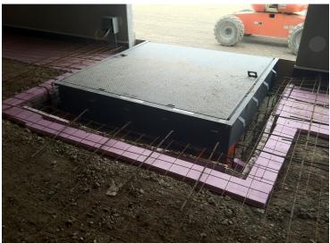
The dock leveler is set onto the pad, positioned and leveled to the finished floor height. The dock leveler is then anchored, using the supplied anchor brackets.
