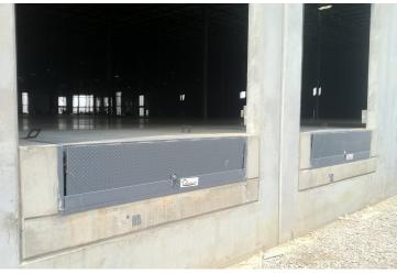
blocked. The concrete is poured in two pours following the manufacturers installation instructions.
