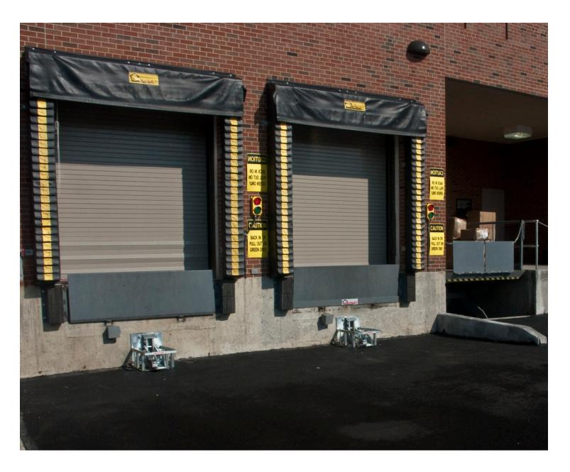
The use of the elevating dock lift in combination with a conventional dock leveler is more cost effective than a combination dock leveler and lift. It reduces maintenance and provides maximum flexibility in the trucks / trailers that can be serviced as well as providing the abilty of the lift truck to be lowered for use on the outside driveway.
