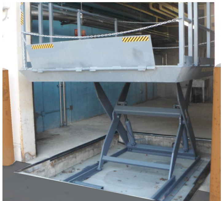
Exterior view of new unit with dual cylinders
