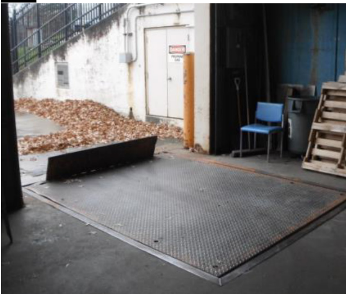
Original dock lift in closed position
