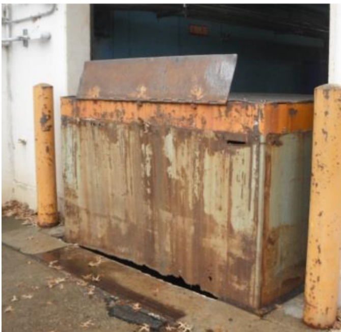
Exterior view of original unit
